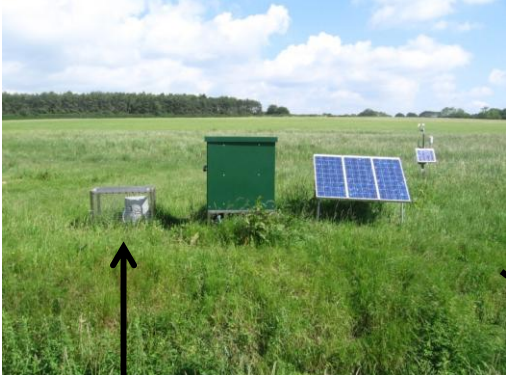
Extra ISCOs installed
